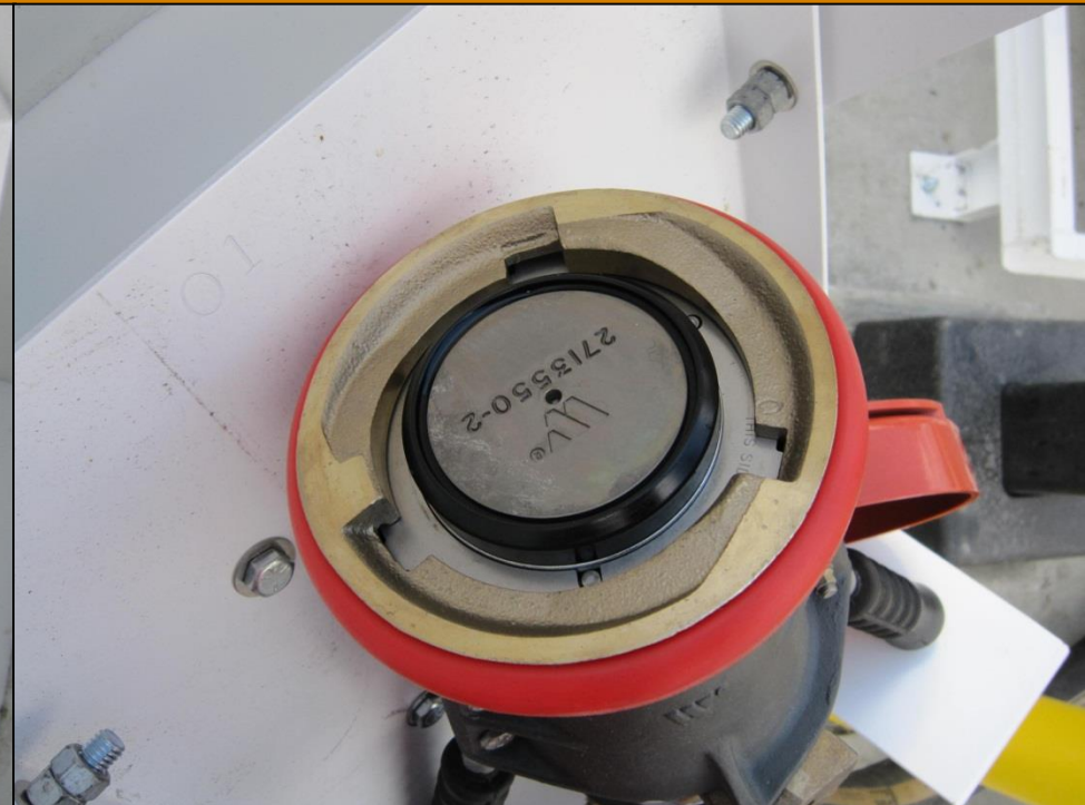
Loading Station Jet A Dry Break Coupler
