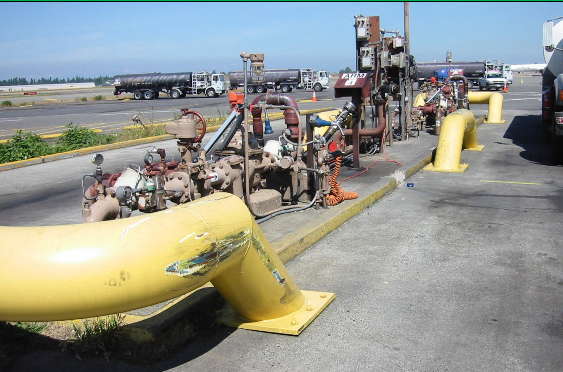
This loading station is protected against physical damage by ground vehicles.
