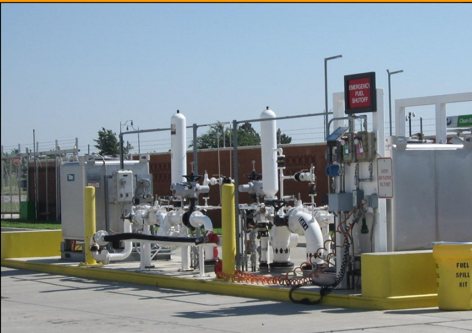
Emergency Fuel Shutoff for Loading Station
