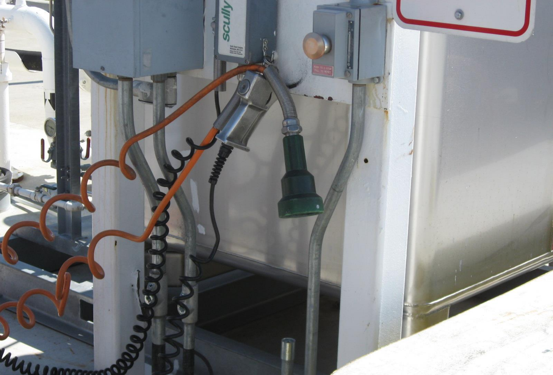
Some fuel loading facilities are equipped with a Scully system, which incorporates both the deadman and bonding features into the system.
