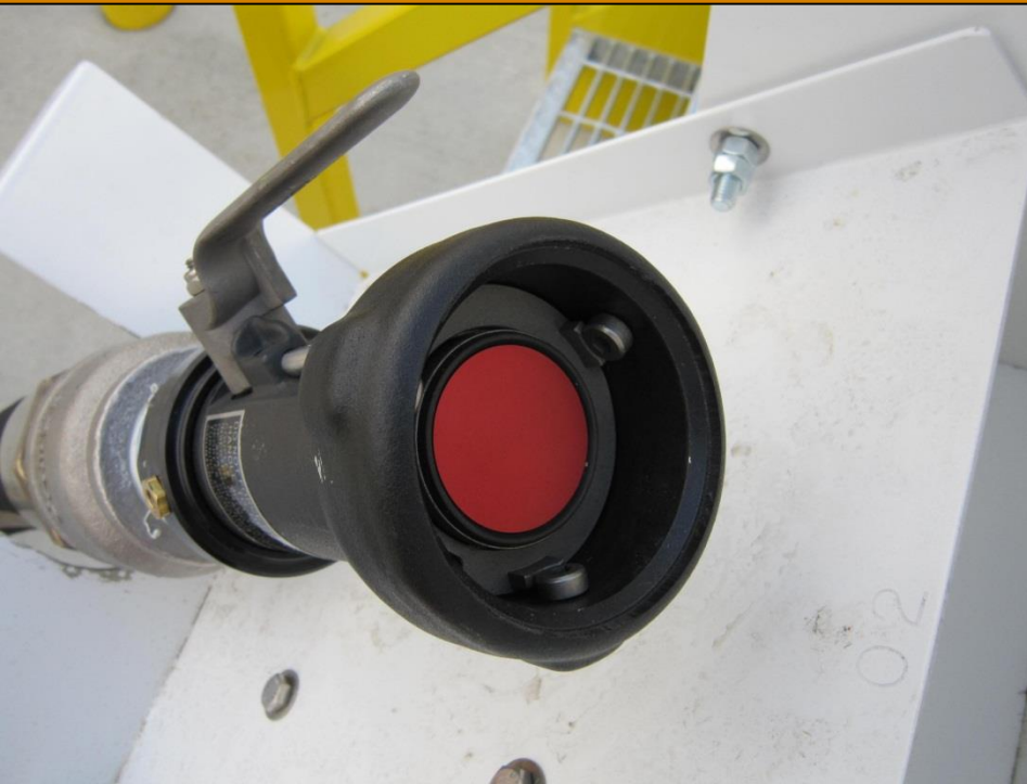
Loading Station 100LL Dry Break Coupler
